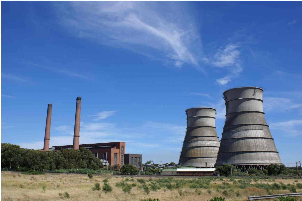
Disused coal factory in Cape Town, South Africa. Its dismantling is intended to make way for new modes of energy. Credit : DanielVDM
