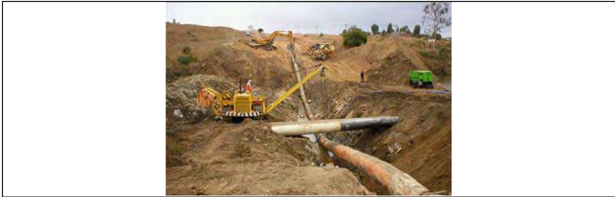
Figure 9. Open-cut pipeline crossing, horizontal pipes above pipeline for water flow 101
