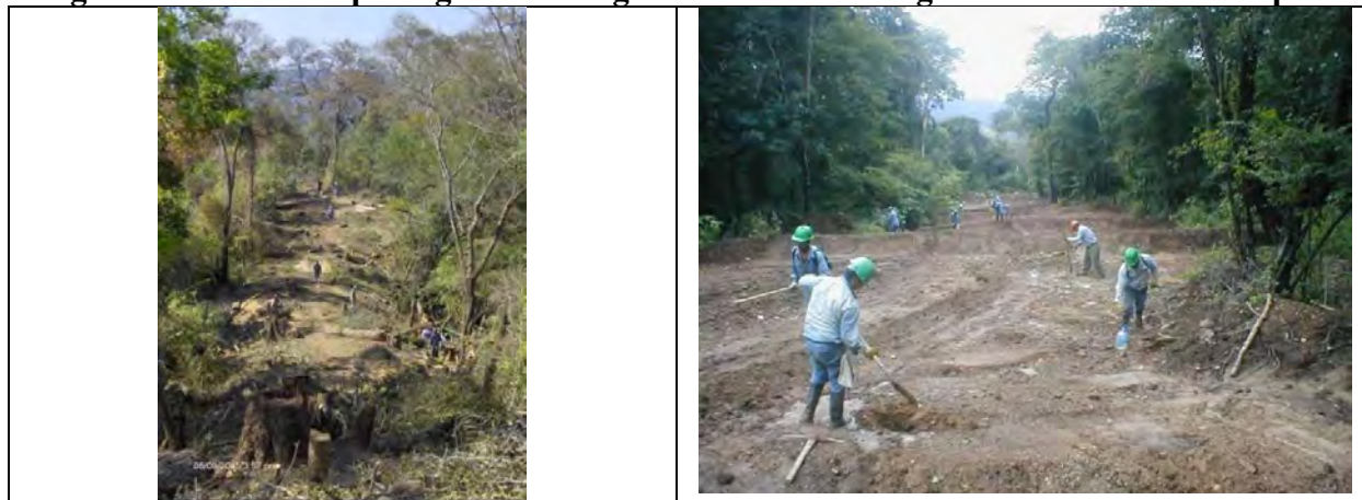
Figures 5a and 5b. Opening and closing narrow ROW using labor intensive technique 96
