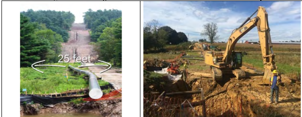
Figures 6a and 6b. Typical Pennsylvania 15-meter pipeline RoW (25 feet on either side of centerline), 97 and clearing of RoW for 20-inch diameter Mariner East Pipeline 98
